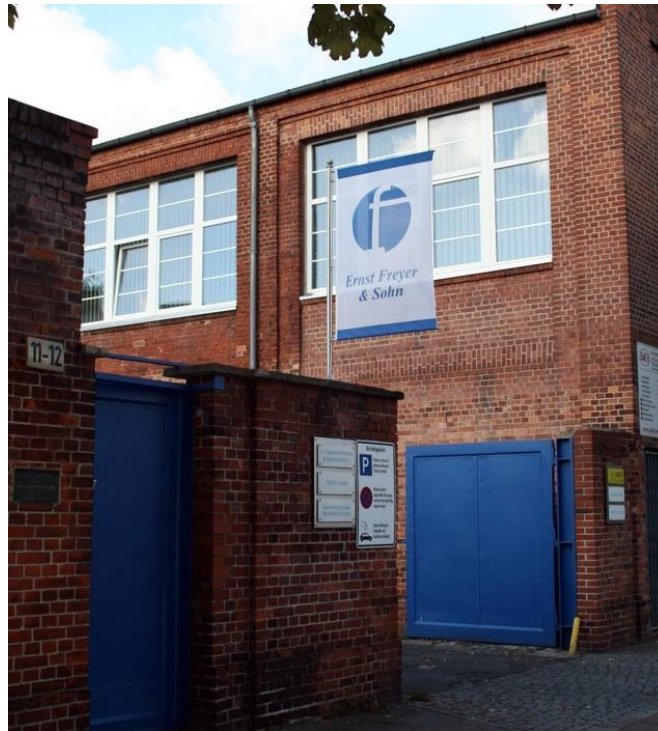
Figure 3. Case Study 3 – Industrial / Tertiary building, Berlin, Germany
