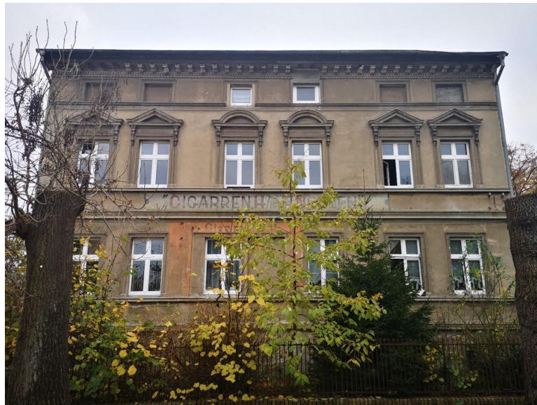
Figure 2. Case Study 2 - Residential/ Multi-family building, Velten, Germany.
