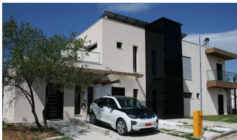
Figure 1. Case Study 1 - nZEB Smart House DIH, Thessaloniki, Greece
